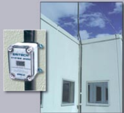
The ERITECH System 3000 ERICORE downconductor is easily retro-fitted to existing structures. Inset: ERITECH Lightning Event Counter (LEC IV) installed to register strikes to System 3000.
